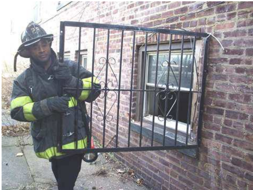
As mentioned earlier, focus your efforts on one side and pull the security bar assembly away from the building.
