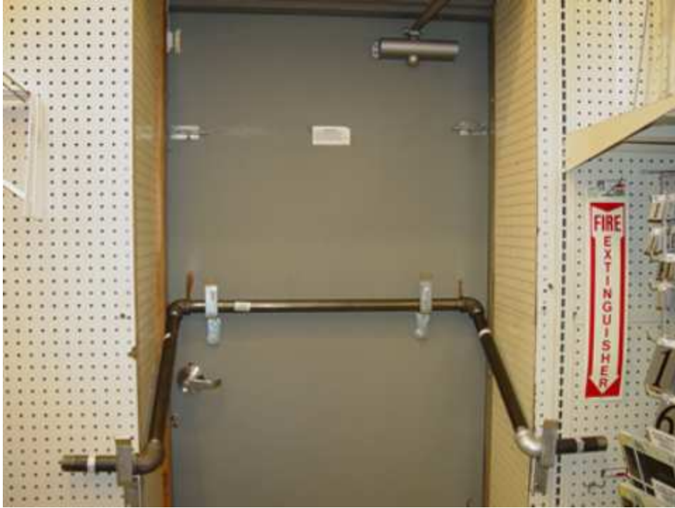
Here's a shot of the entire installation.
